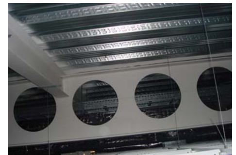
Figure 3: Primary and secondary beams supporting trapezoidal steel decking for RC slab
