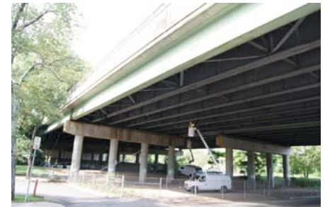
Figure 2: Bridge support, main girders and means of access.
