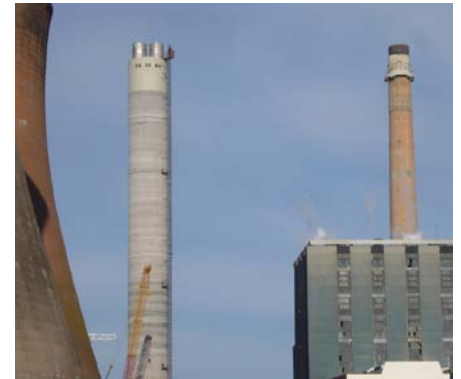
Figure 1: Tandem chimneys at Rugeley Power Station
